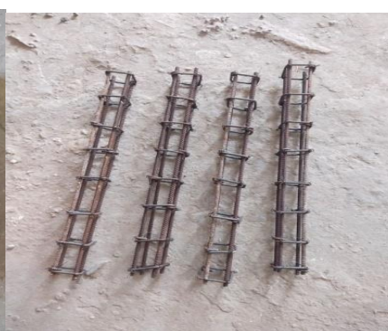
Fig 6: Reinforcement preparation
