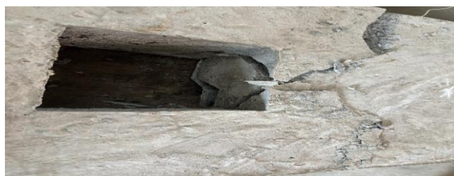
Fig 12. Crack Near Opening
